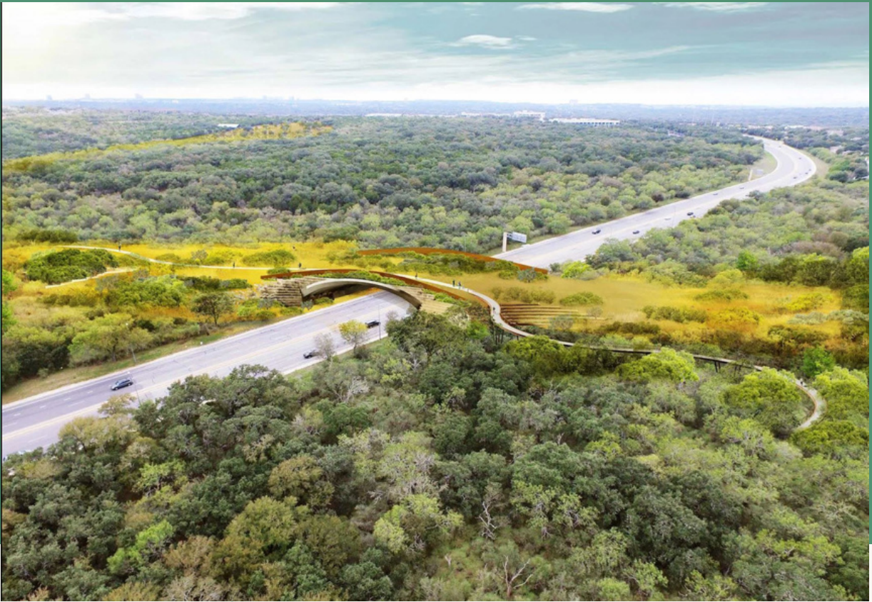
Phil Hardberger Land Bridge ( City of San Antonio, 2022 )
